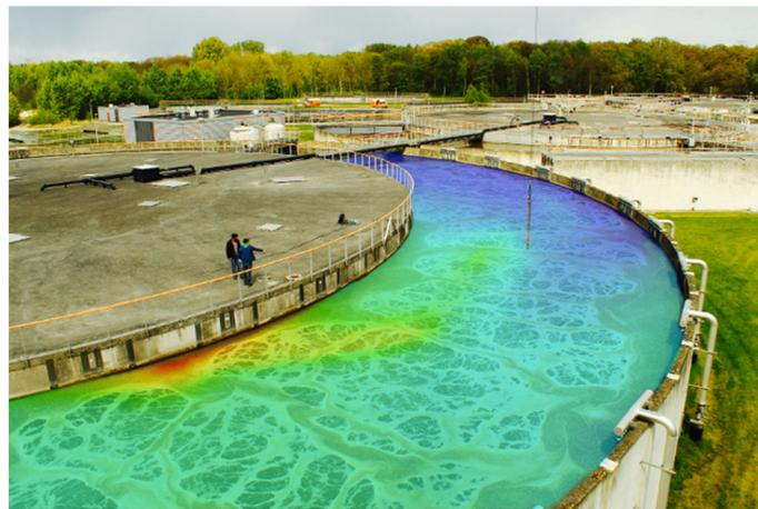
Figure 1 – The Eindhoven WWTP, with an overlay of CFD simulation of air distribution
